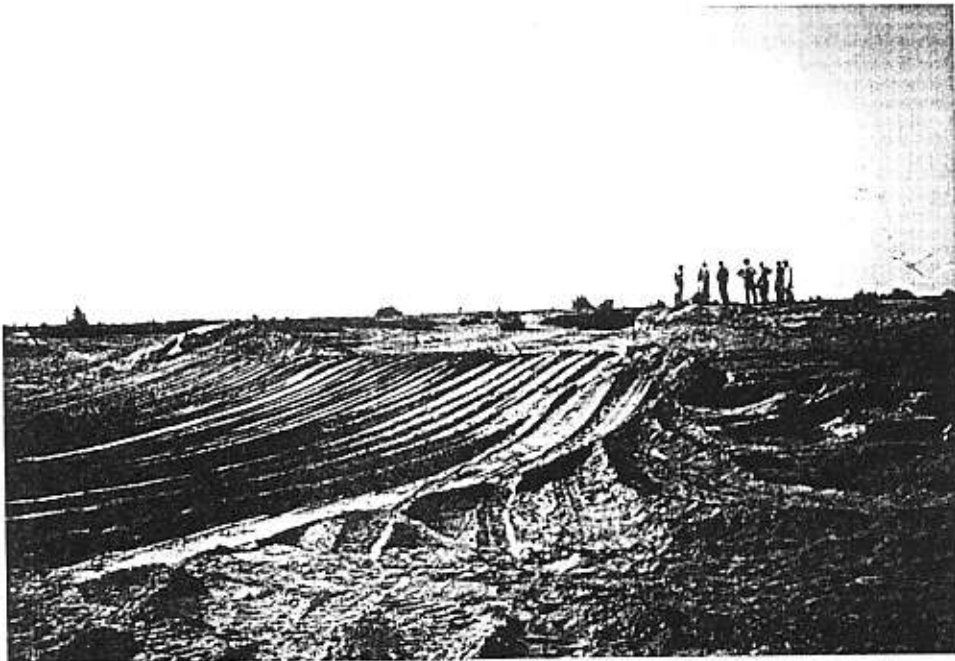
PHOTO 18: JAMAK BUND UNDER CONSTRUCTION
