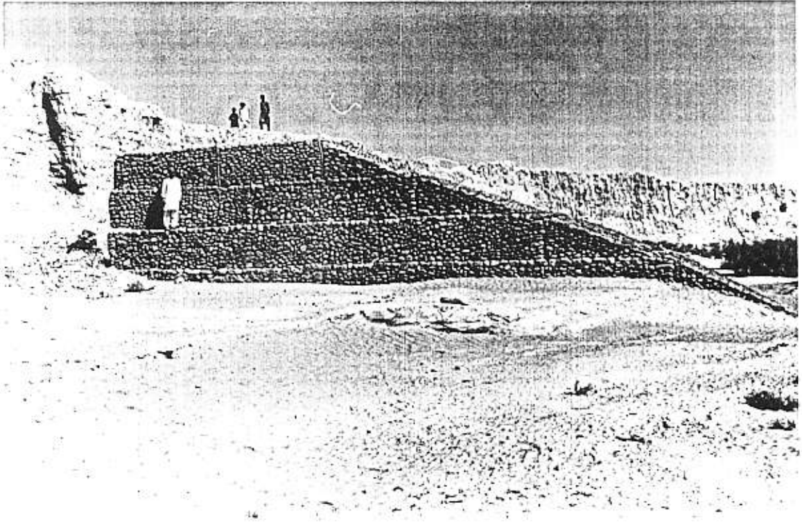
PHOTO 3: GABION SPUR, BUILT BY IRRIGATION DEPARTMENT, NEAR SHAYAN VILLAGE
